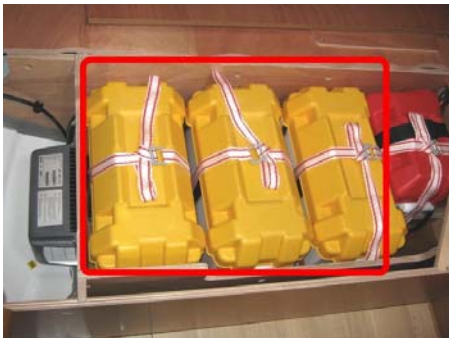
Service batteries: 3 x 115A Location: Starboard aft cabin
