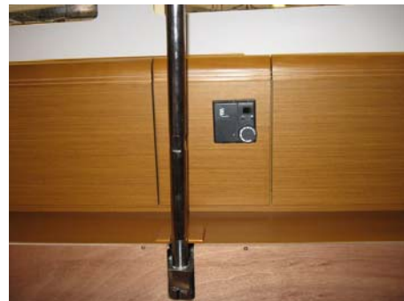
Control - Heating unit
