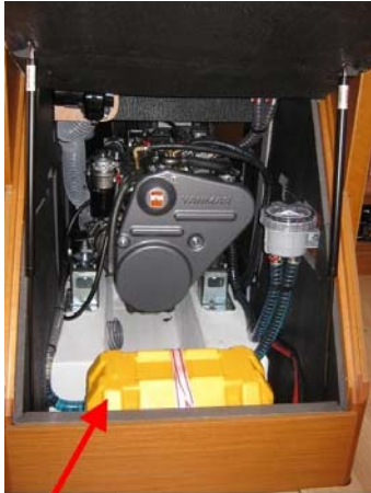
Engine battery: 110A Location: Companionway
