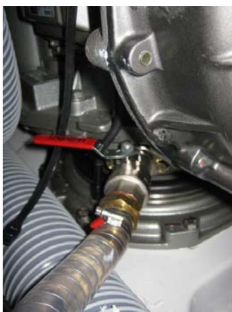
Engine water intake valve: Located directly on the saildrive
