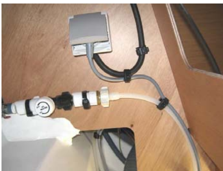
Supply valve House water / Dishwasher
