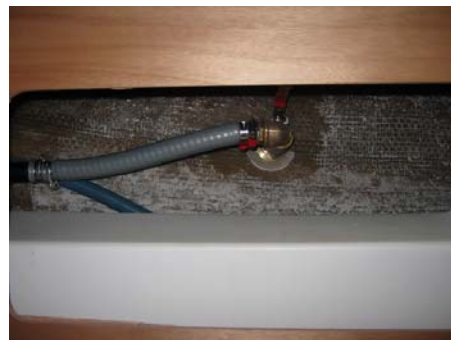
Washing machine outlet
