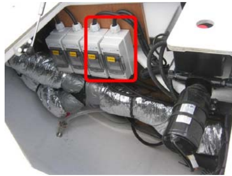
Circuit breakers: Shore / Generator Access: Cockpit locker
