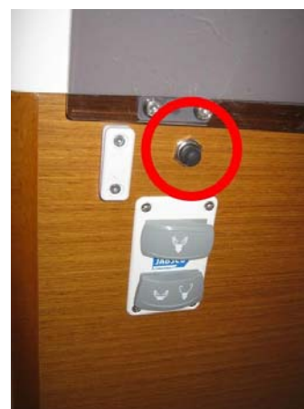
Control - Draining pump for shower
