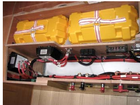
Spare service batteries: 2 x 115A Location: Port aft cabin
