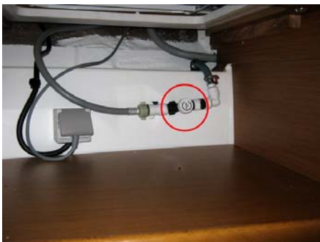
Supply valve House water / Washer
