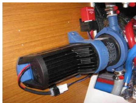
Control - Draining pump for shower
