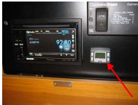
Ref 5: Control - Heating
